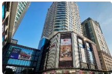
Ba Trieu Office Building
